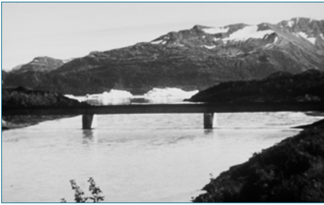
Figure 17–9. Glulam beam bridge over the Dangerous River, near Yukatat, Alaska, consists of three 43.5-m (143-ft) spans. Each span is supported by four 2.3-m (91.5-in.-) deep glulam beams.
