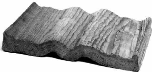
Figure 13-10. Severe collapse in western redcedar.
